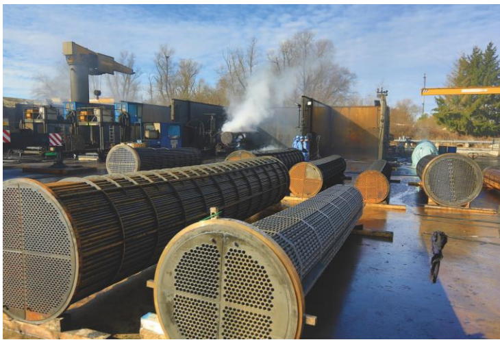
Image 2 Example of a bundle cleaning spray site
