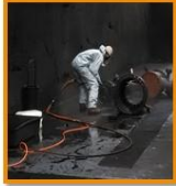
A) Trillingsbelasting (bv nozzle)
